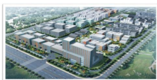
Chengdu Base (under construction )
