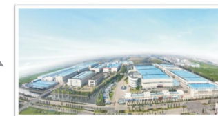
Ningbo Base (Air-Con、Power、Hospital)
