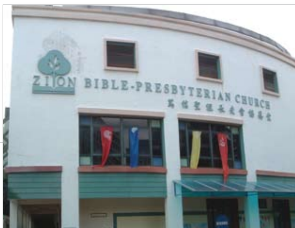
Zion Church, Singapore Commercial Sector Indoor Type: Ceiling Concealed, Ceiling Convertible and Ceiling Cassette
