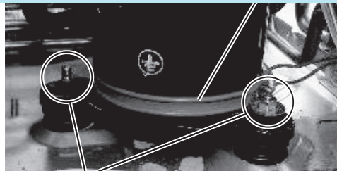
Nut of compressor fixing bolts
